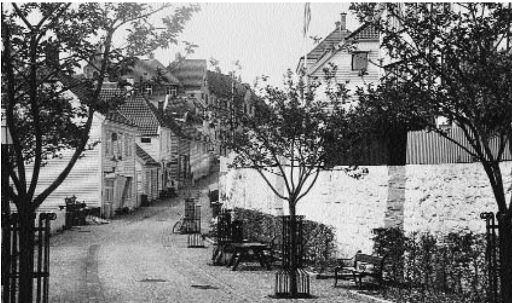
Figure 5.66 Old Bergen, traffic calming.
