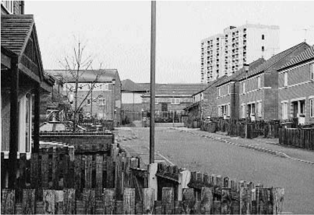
Figure 3.2 Radford. A return to a street architecture after demolition of 1960s deck access flats.
