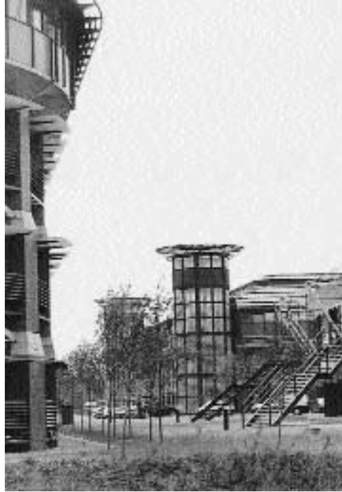
Figure 4.12 Canalside development, Nottingham: The Inland Revenue Building by Michael Hopkins and Partners.
