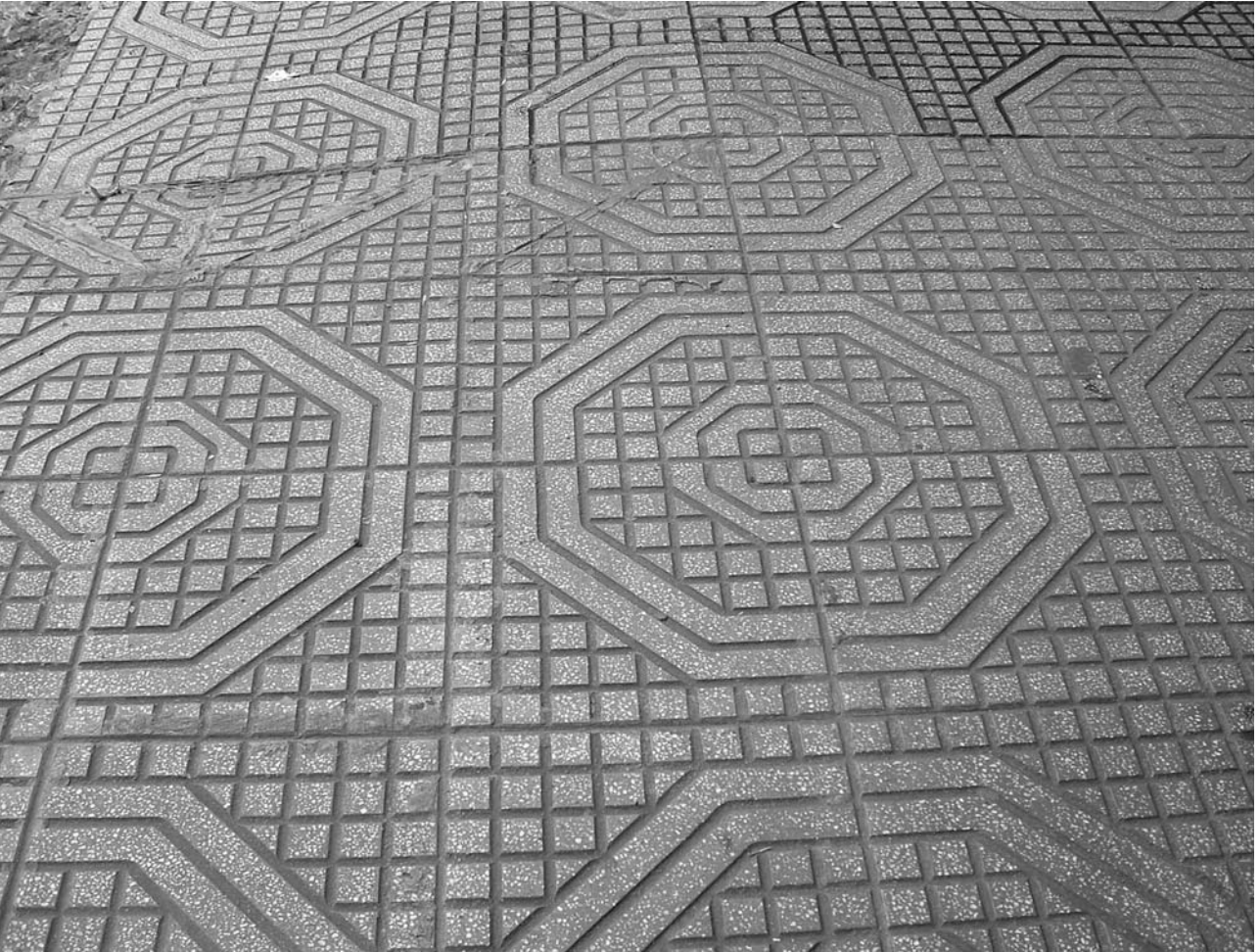
Figure 9.6 The rough surface of this paving can be difficult for older people and others with mobility problems to walk on. The pattern is likely to cause dizziness and confusion in people with visual and cognitive impairments.
