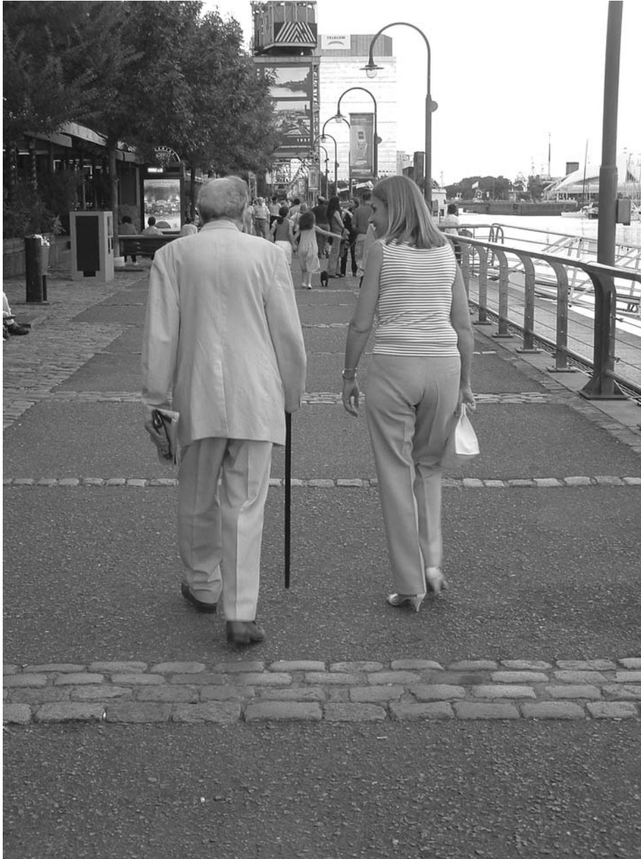
Figure 9.5 These cobbled strips are a trip hazard – not only are they slightly raised but they will look like steps to people with impaired depth perception.
