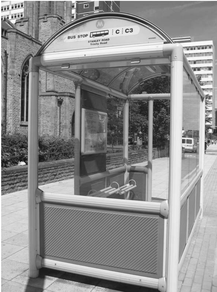
Figure 8.6 Older people prefer enclosed bus shelters with seating and transparent sides or large windows. (Photograph by SURFACE Inclusive Design Research Centre.)
