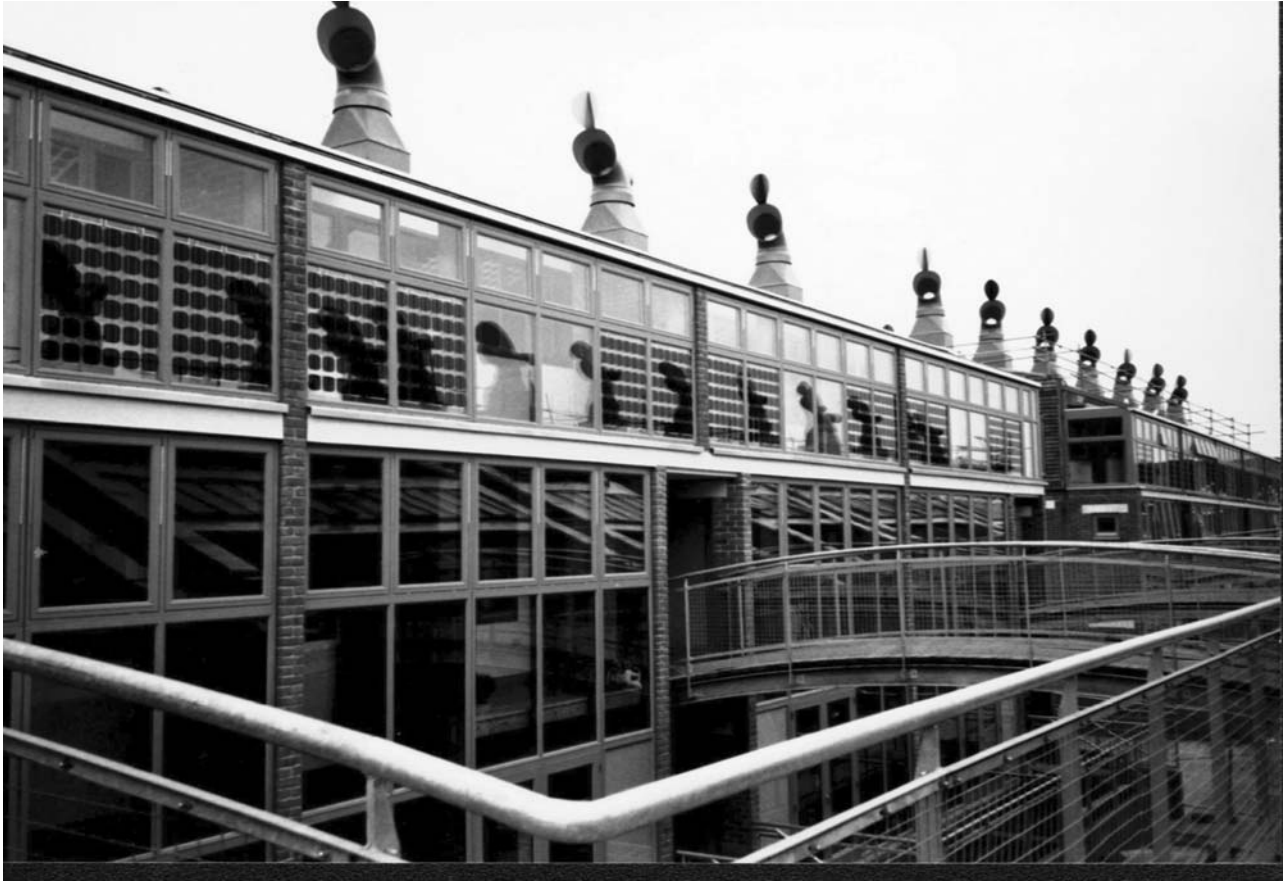
Figure 1.3 BedZED, Sutton: one of the new sustainable developments in the UK. (Photograph by Carol Dair.)
